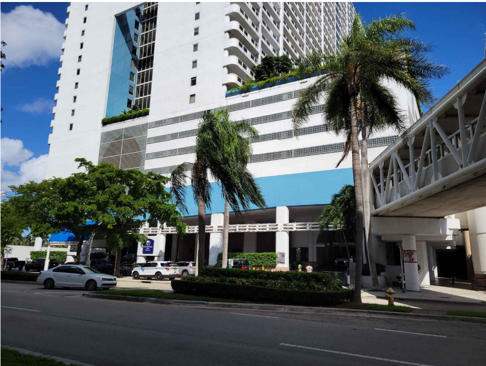
Existing Site Photograph
