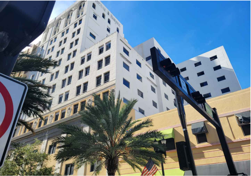
Existing Site Photograph
