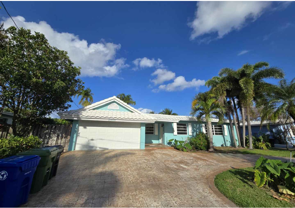
Existing Site Photograph
