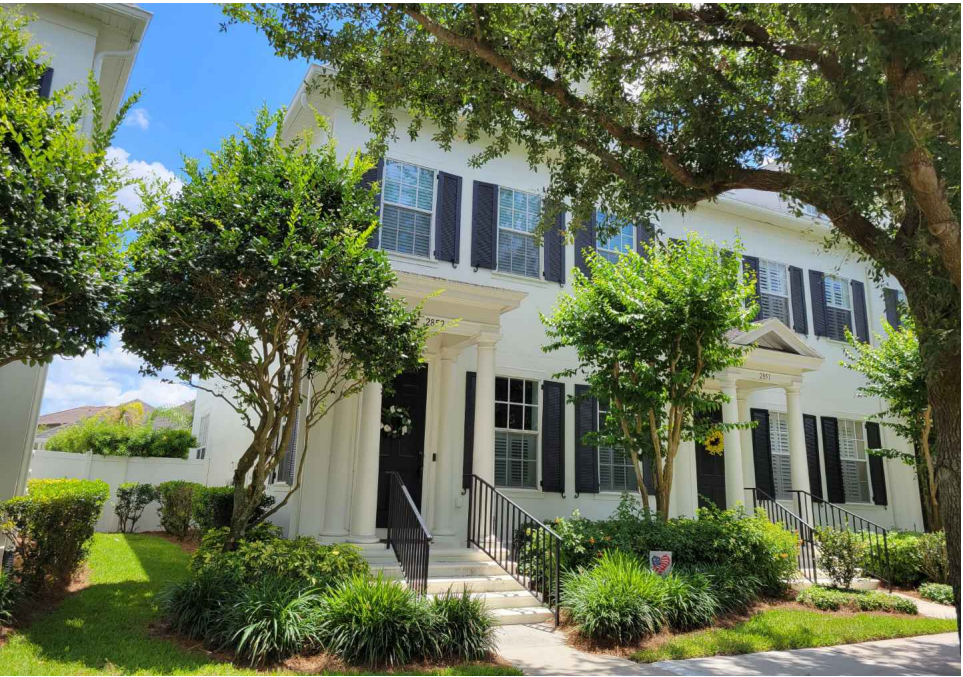
Existing Site Photograph
